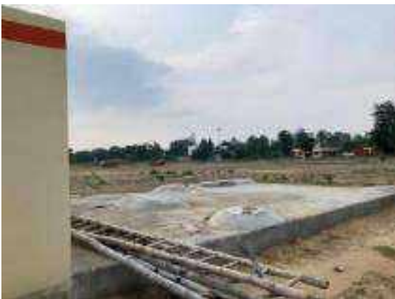
Static Water Tank West Campus
