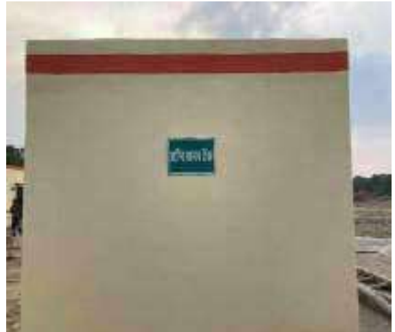
Fire Fighting Water Tank West Campus
