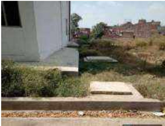
RWH Pits East Campus
