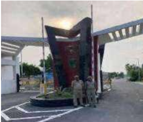
Main Gate West Campus Security
