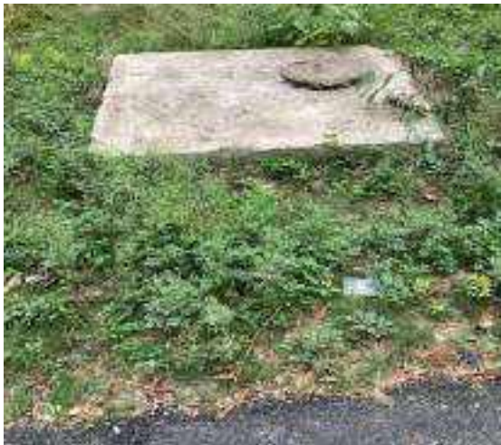
RWH Pit West Campus
