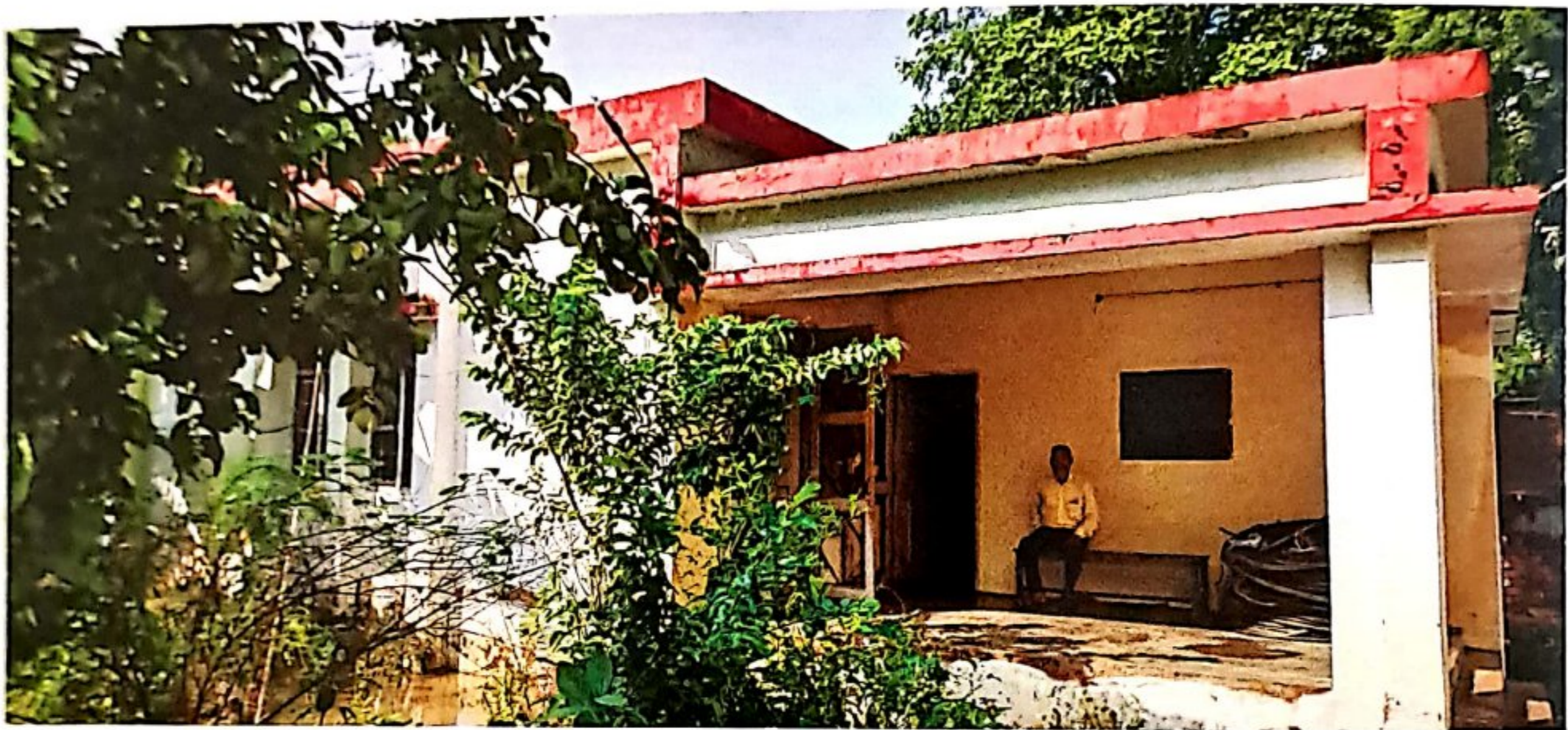
Office building of Electrical Sub-station
