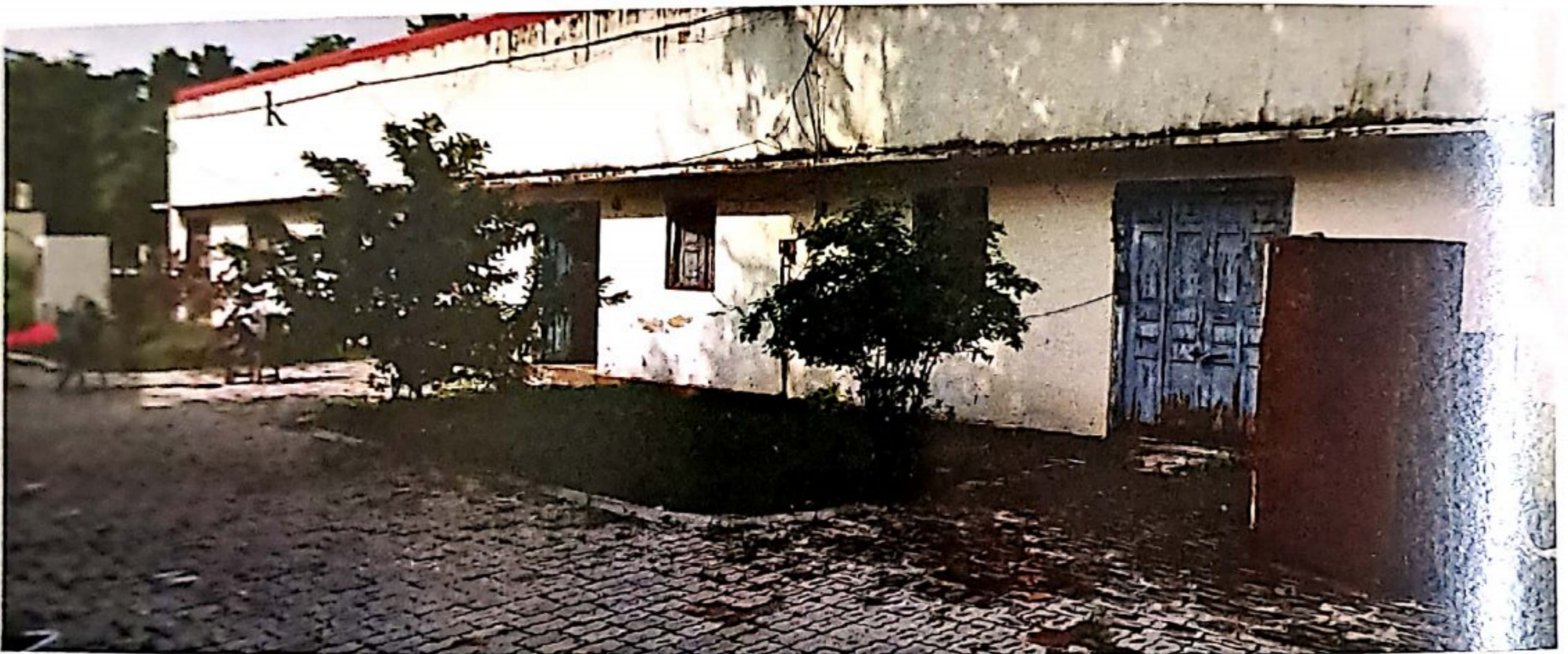
Mechanical Maintenance Section Building
