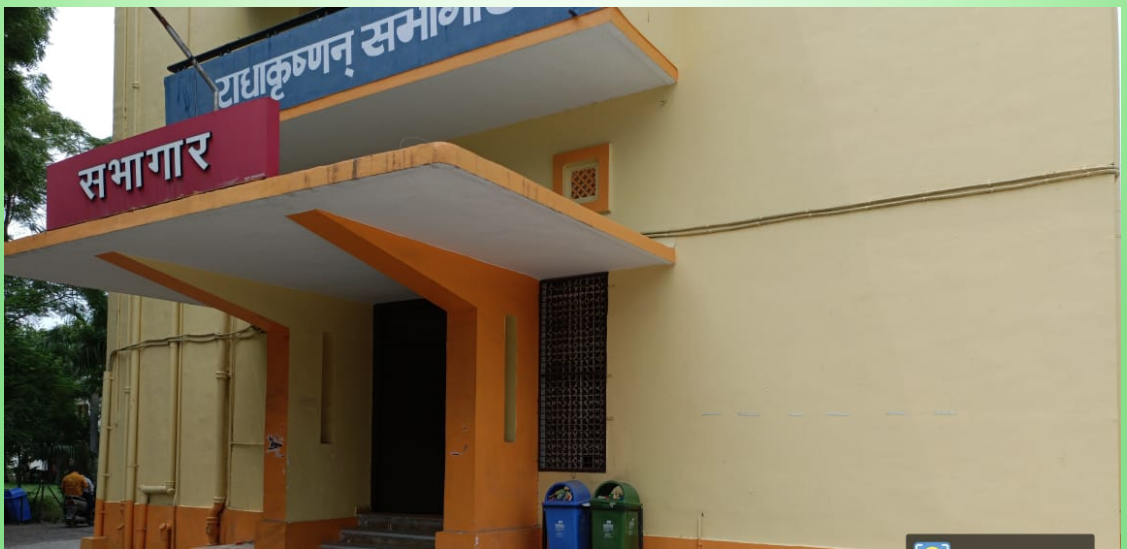
Waste Collection Bins Outside Auditorium
