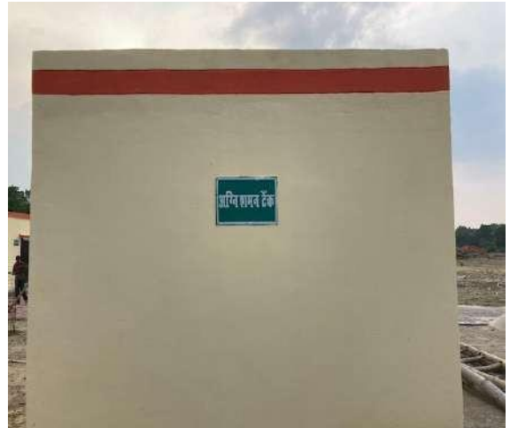
Fire Fighting Water Tank West Campus
