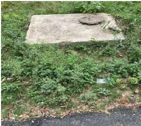
RWH Pit West Campus
