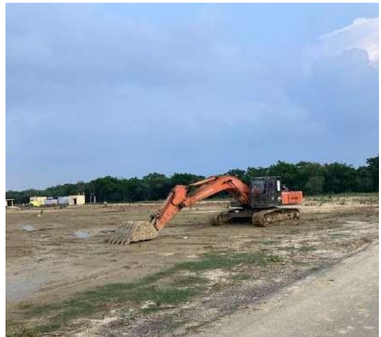
Preparing Ground for New Garden Area West Campus
