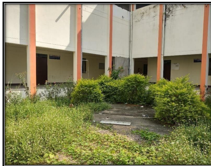
RWH Near Classrooms (G1 to G7)
