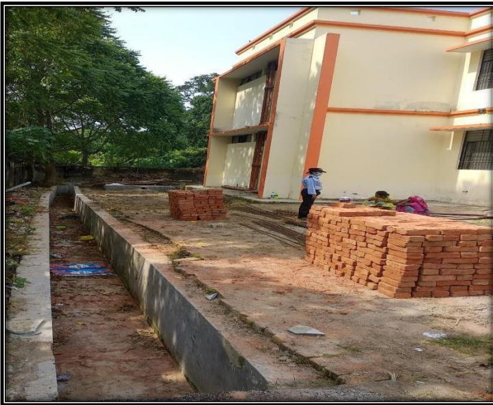
Storm Water Drain in New GH-III
