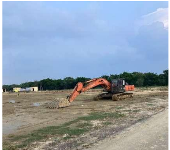
Preparing Ground for New Garden Area West Campus
