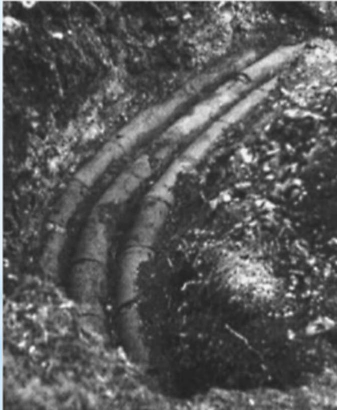
From 283 to 133 BC, they built a series of pressurized lead and clay pipelines, up to 45 km long that operated at pressures exceeding 1.7 MPa (180 m of head)
